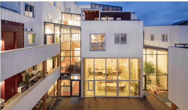
Fig. 15. The exterior of the “allrom”. (Photograph by Helen & Hard, Vindmøllebakken , Arkitektfirma Helen & Hard AS).
